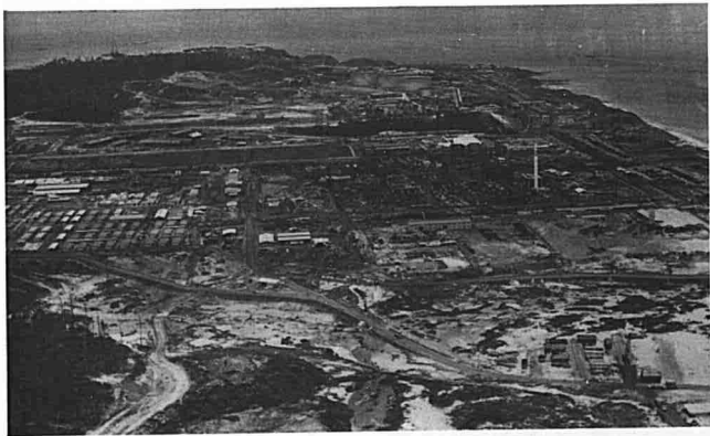
Tanjung Kidurong, the new industrial area and port near Bintulu.
