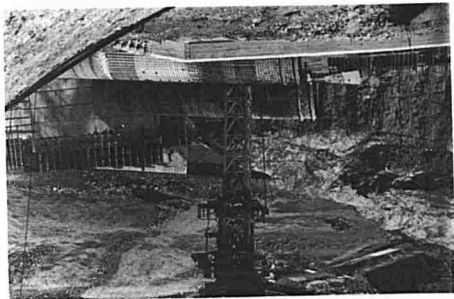
Constructing the main dam at the Batang Ai Hydroelectric Project.
