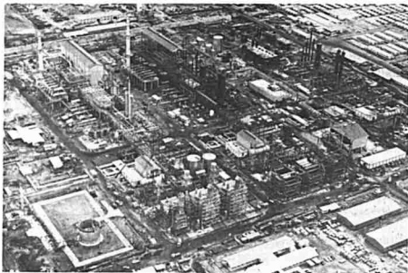
The Liquefied Natural Gas (LNG) Plant in Bintulu.
